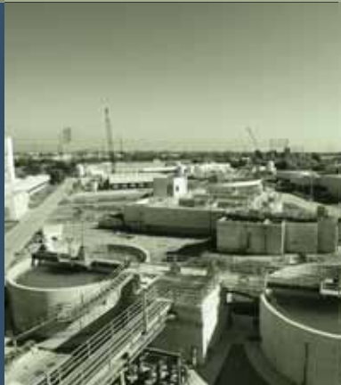
HDR, as a part of the Design-Build joint venture, executed the West Basin $ 52 Million Design-Build Water Reclamation Plant Project meeting challenging work conditions successfully.
