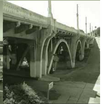
HDR worked closely with Caltrans Structures Local Assistance during the analysis and retrofit strategy phase.
